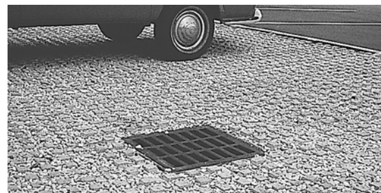
Figure 18. Concrete grids with aggregate in the openings
