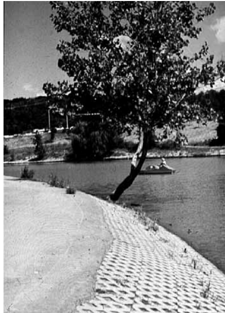
Figure 4. Lakeside stabilization
