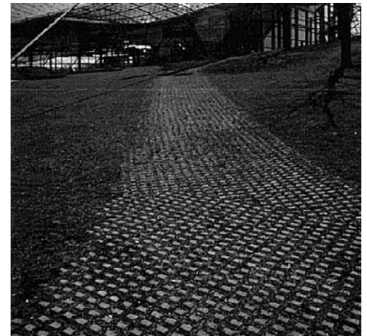
Figure 7. Service access lane
